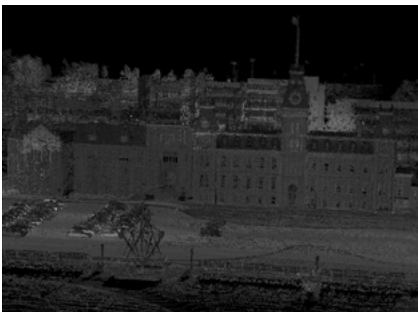
LIDAR scan of buildings on the campus of the Royal Military College, Kingston, acquired by the TITAN system in May, 2007. In LIDAR, the point of view of a scene such as this is not the point from which the scanner collected the data - in this case, along the roadways.
